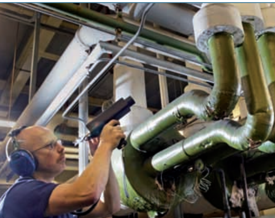
Above: Eriks' engineers survey for air leaks Right: An Olympus Iplex MX videoscope, used by Veolia to survey packing material in a cooling tower
